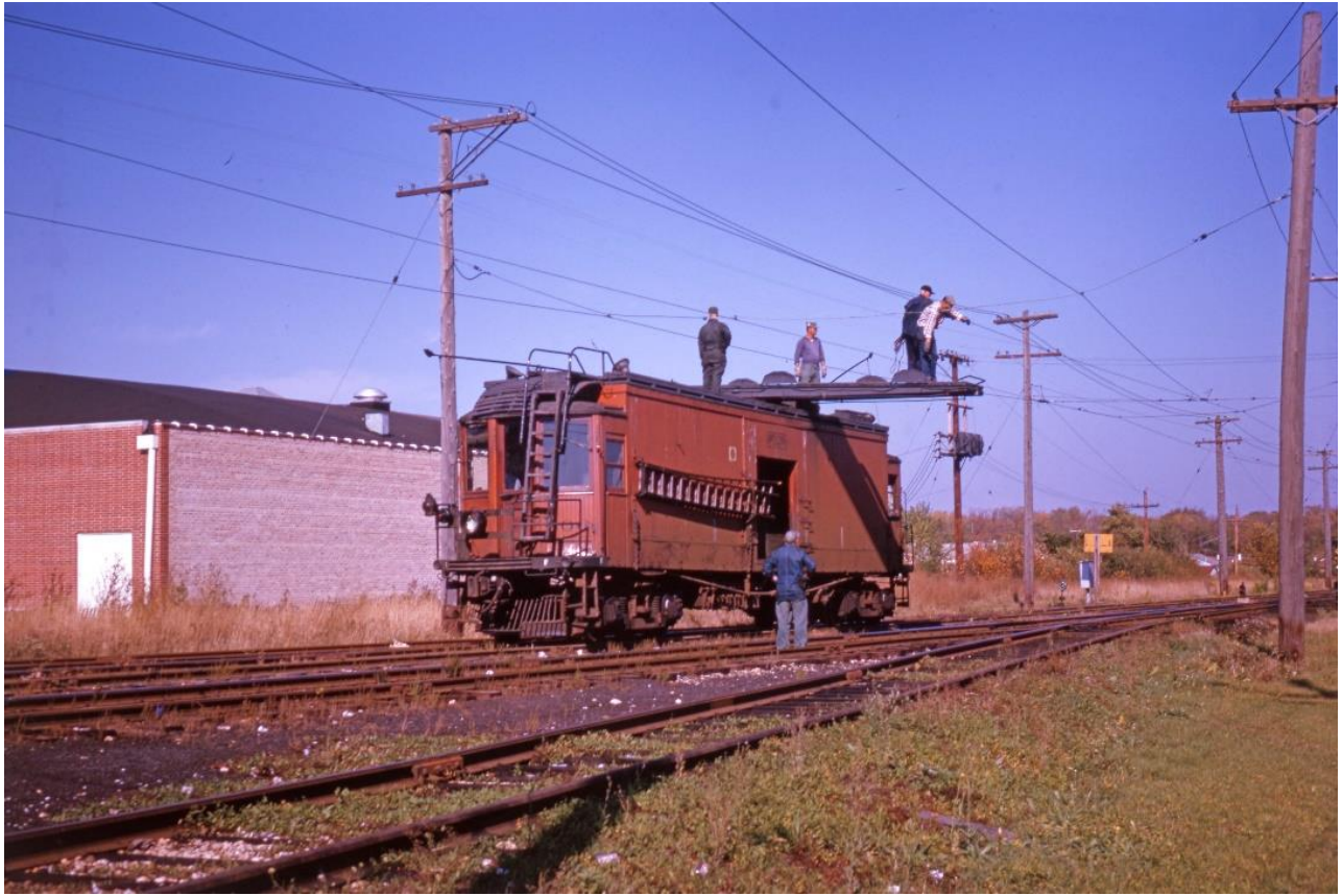
Nearing the end of its service on CNS&M, the line crew is at work at Mundelein, Illinois, on 10 October 1962. The movable platform is necessary when working on adjacent tracks.
