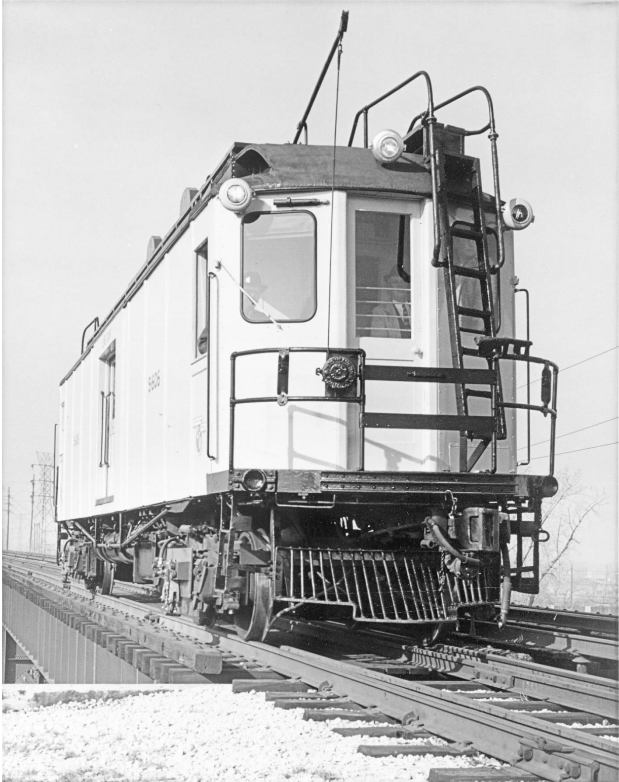
Rebuilt by the Chicago Transit Authority (CTA) in 1964, tower car #S-606 is posed at McCormick Boulevard in Skokie on its inaugural run. While owned by CTA, tower car #S-606 served its original CNS&M home trackage in Skokie, as well the former Milwaukee Road Wilmette Branch freight and passenger trackage.
