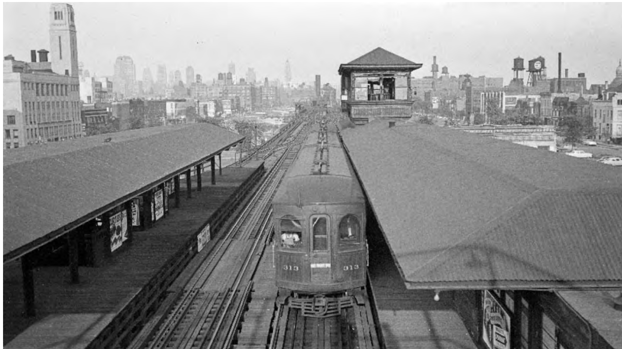
Sunset Lines car #313, Marshfield Avenue, Chicago, 21 August 1953. Interurban cars that operated over Chicago's 'L' were constrained by everything seen and unseen in this view. The pedestrian bridge that served as the photographer's perch limited the height of these cars.
