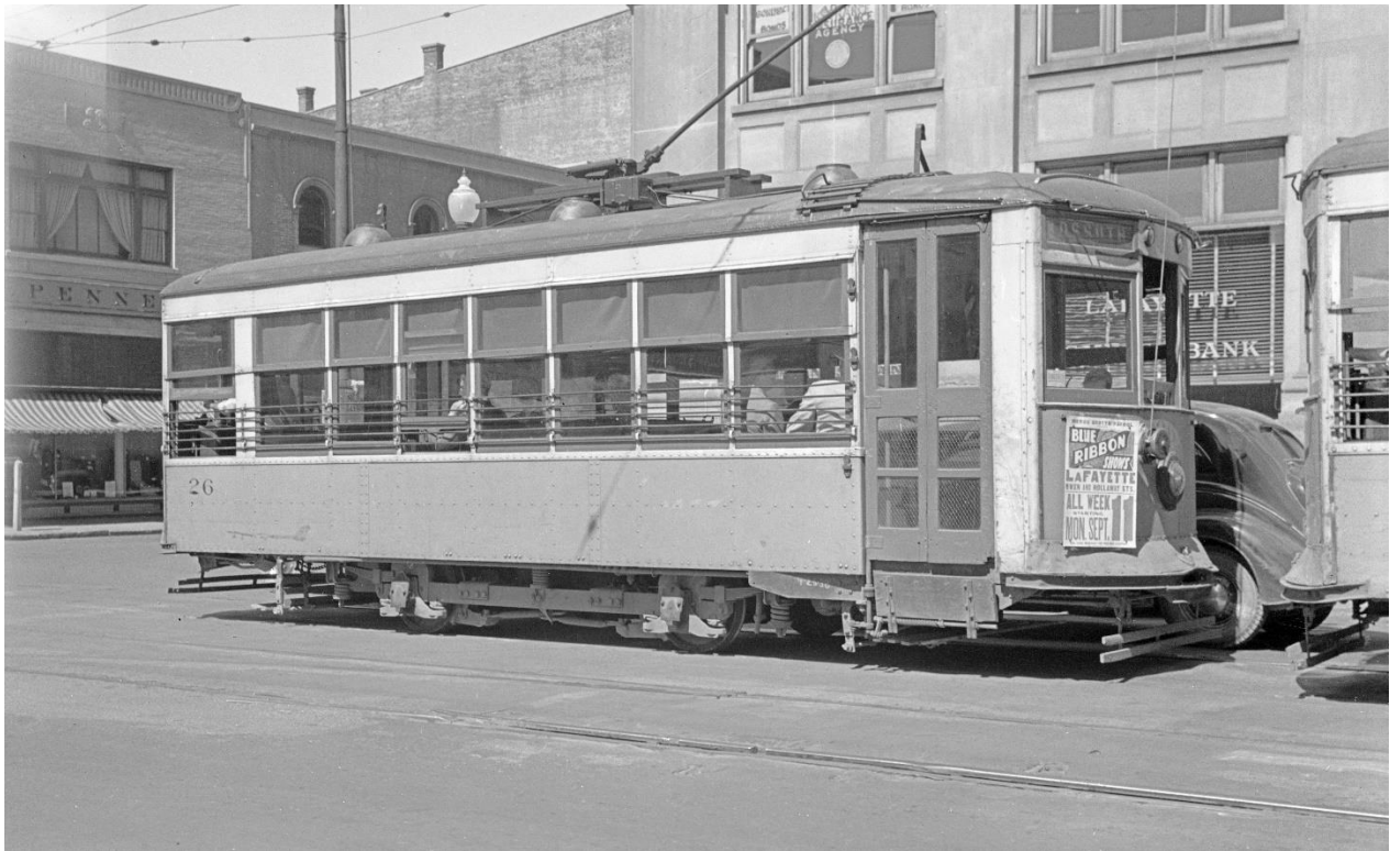
Lafayette Street Railway Birney Streetcar at Main and Third streets, 1939. Birneys were hard-riding, noisy cars.
