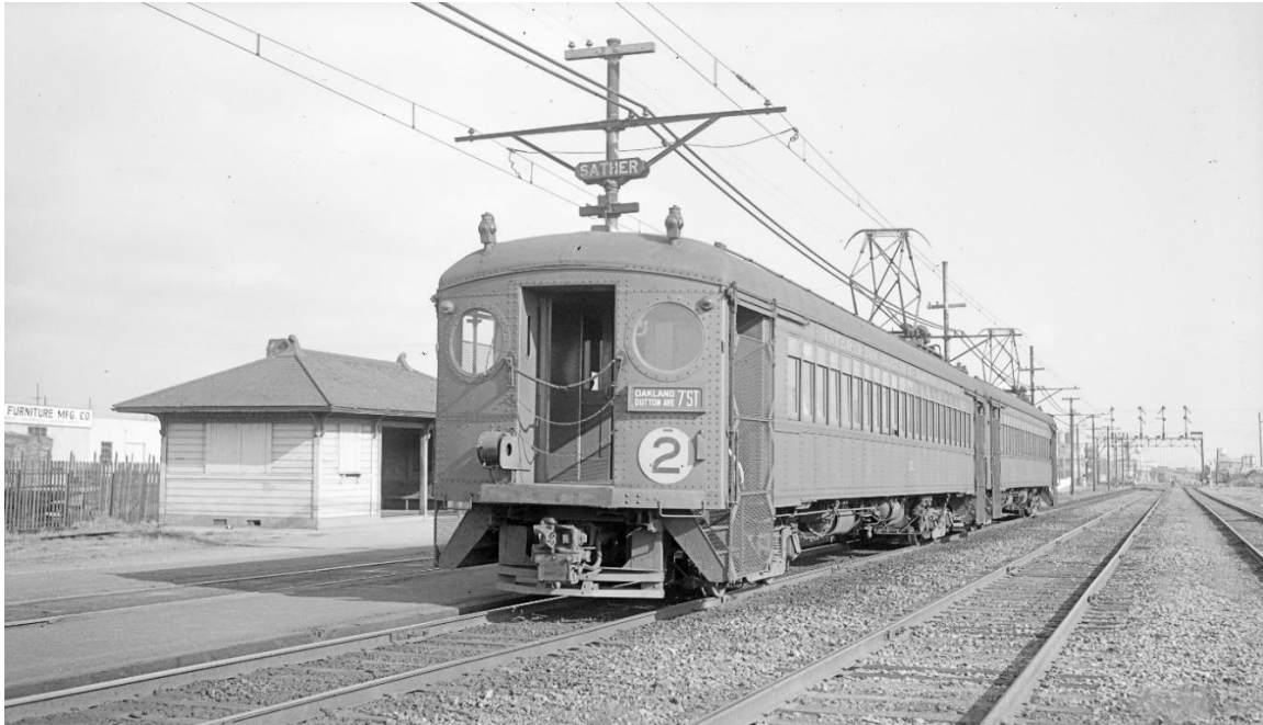
The East Bay suburban services of the Southern Pacific (SP) were electrified in 1911 with a fleet that reached 174 cars after subsequent orders of identical cars were received as late as 1924. These motorized coaches seated 116. Oakland, California, 1940.
