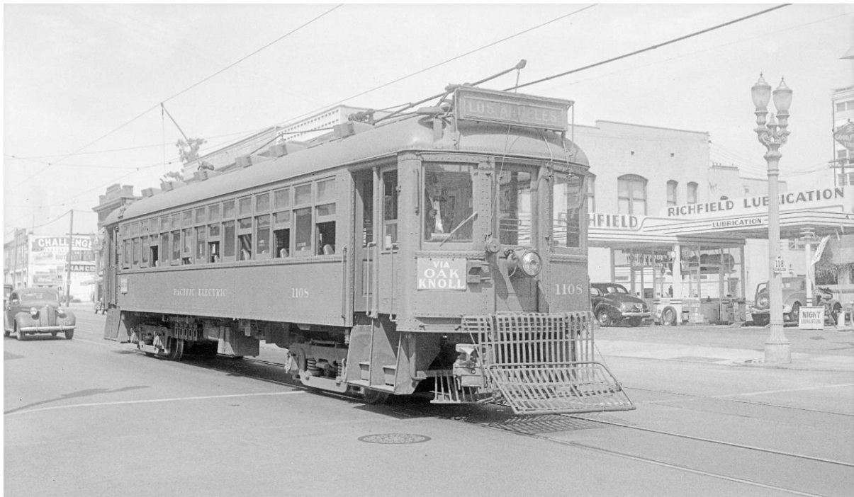
Steel roofs prevailed across all classes of steam railroad equipment including the interurban and suburban cars of the Southern Pacific. Pacific Electric car #1108, 31 August 1941. (Photographer credit: Victor Vinzent DuBrutz).
