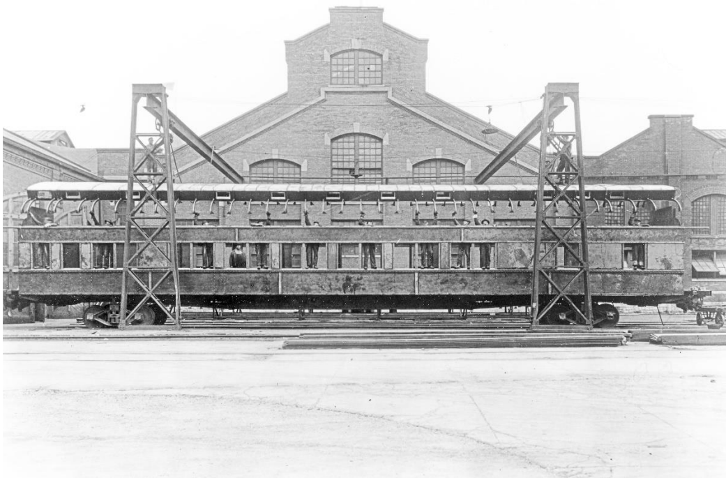
Next, the roof was lowered and riveted to the side structure. Pullman, Illinois, circa 1922.
