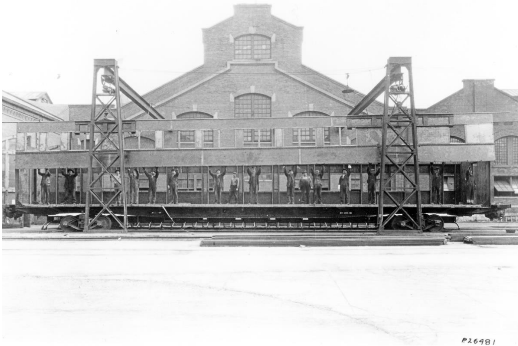
Car side being lowered onto an underframe. Because the sides of the car were non-structural, they were lowered onto the trapezoidal structure and then riveted in place.
