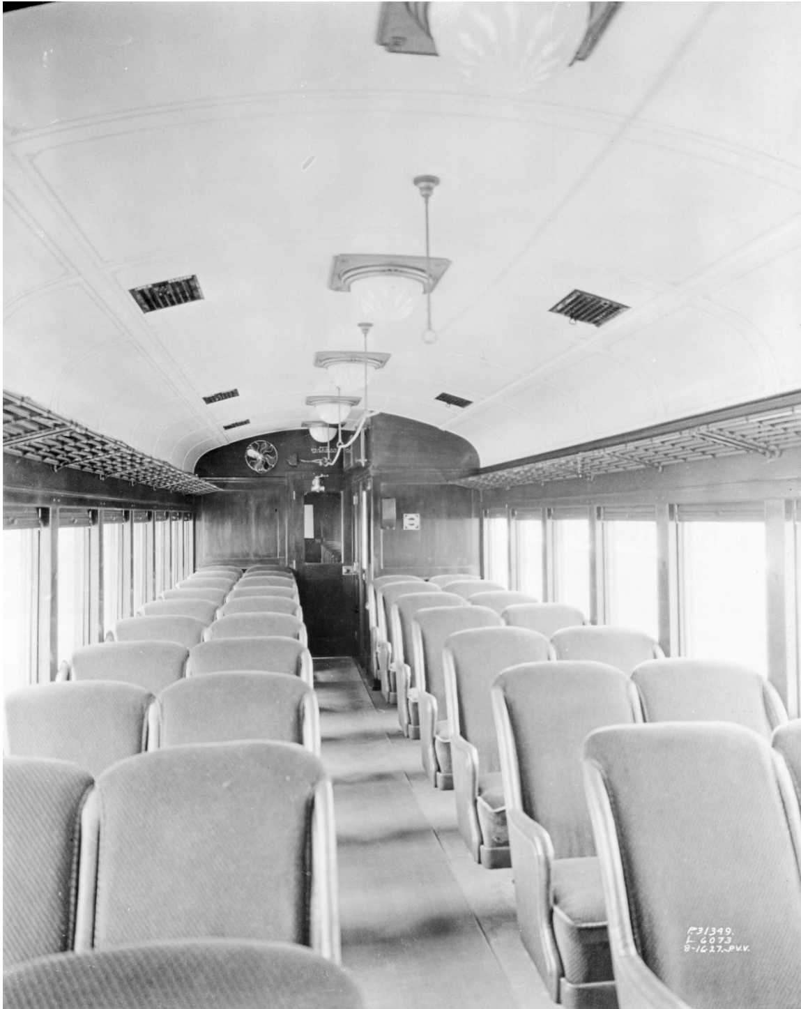
South Shore Line car #21 at Pullman, 16 August 1927. The South Shore Line was slow to adopt bucket seats in light of the trend already underway in the interurban industry. The bucket seats sat on a turntable mechanism. Depressing a foot pedal just below the seat cushion allowed the bucket seats to be turned to face forward. Non-motorized coach trailers were similar but had a single unisex restroom; the motor cars had separate restrooms for men and women. (Photographer credit: John P. Van Vorst for Pullman Car & Manufacturing Company).
