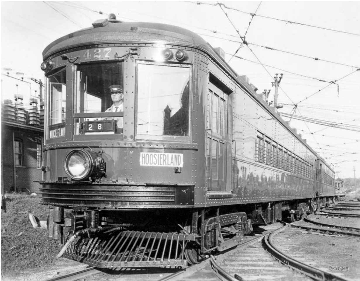
Union Traction heavyweight interurban cars at Anderson, Indiana, 1925. This fleet of cars was bought by Arthur Brady, the receiver for Union Traction. Typical of so-called receivers' cars the interiors were all steel with painted wood-graining to make the cars more appealing.
