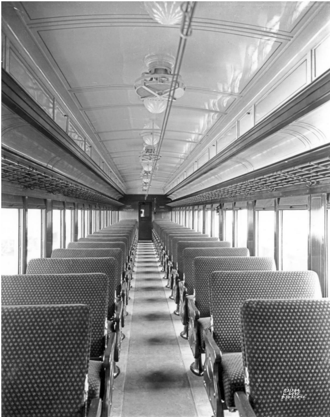
Baltimore and Ohio Railroad car #5315, at Pullman 30 September 1927. Contemporary steam railroad car design was stagnant throughout the 1920s. The walkover seats in this view are of an older design that lacked the back and “head roll” neck support of those in the wooden South Shore Lines coaches of a generation before. The design of steam railroad day coaches was a full decade behind the design standards of the interurbans. 59 But the steam railroads ignored the impact of the automobile at their own peril. (Photographer credit: John P. Van Vorst for Pullman Car & Manufacturing Company).
