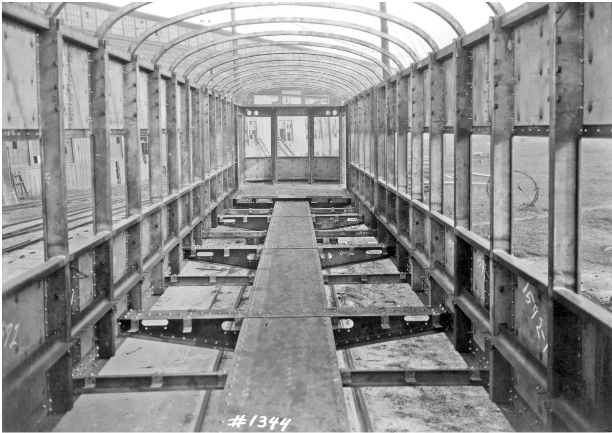
Union Traction car #431, completed framing, St. Louis Car Company, November 1925. This view toward the front of the car shows the pressed-steel floor frame members, U-channel window posts extending from the bottom of the side sills to the top sill, and the pressed steel carlines used to support the wood roof. Typical of a truss-side framed car, nearly all the structural strength is in the floor and sides. (Image Courtesy of the John W. Barriger III National Railroad Library).
