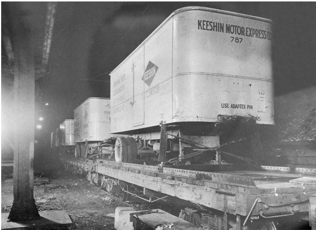
Keeshin Motor Express Company trailers aboard North Shore Line flat cars at the Montrose ramp, Chicago. Keeshin Motor Express was a pioneering trucking company in its use of railroad piggyback services. The technologies developed by the interurbans of the Insull Group made Keeshin's transition from driver-operated hauls to more economic steam railroad piggyback hauls possible.
