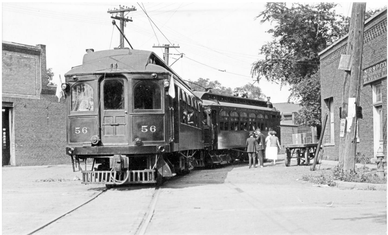
Southern Illinois Railway & Power Company coach-baggage car #56 at Eldorado, Illinois. The carton on the baggage cart at the right is typical of what could be carried in an interurban baggage compartment. Carrying LCL freight added little revenue to a passenger run but did so with virtually no added fixed or variable expense.
